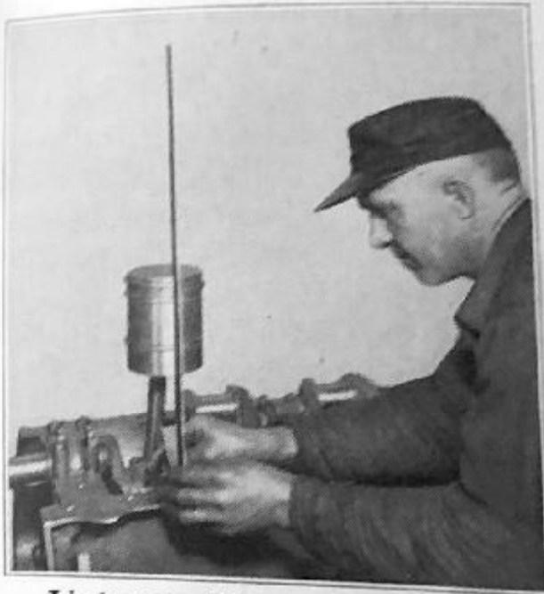
Lining up Pistons with Steel Square at Side
