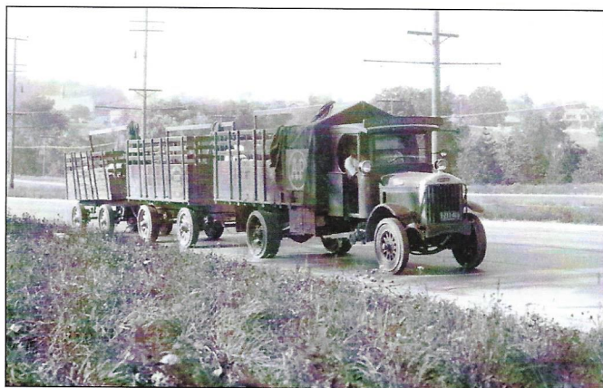
The 2½-ton Gotfredson Model 50 shown in 1928 on famed Woodward Avenue in Bloomfield, Michigan, featured Timken worm drive. A 312-ci Buda ETU 28.9 HP (S.A.E.) engine powered the truck operated by A & P. DPL
